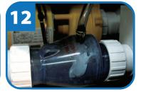
Cascade check valve inside the equipment area, full of water is an indication of no more air in the plumbing line. If the check valve is not full of water, air is still in the plumbing lines.
